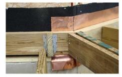
metals in contact with each other will corrode due to galvanic action.
