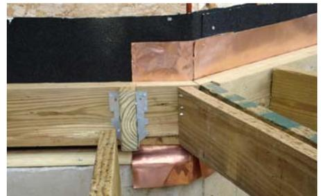
metals in contact with each other will corrode due to galvanic action.
